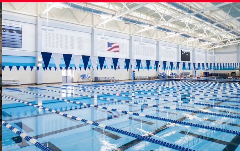
AFTER: LED Westside Aquatic Center Project
